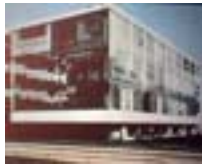
37_Workshop Wing (Shop Block) – Bauhaus – Dessau – 1925 – Gropius
